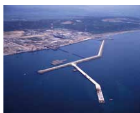
Kashiwazaki-Kariwa Nuclear Power Station
