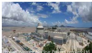
AP1000™ Next Generation Pressurized Water Reactor (Sanmen Nuclear Power Station unit No.1: SNPC)
