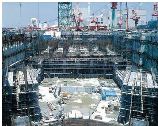
Intake Pond Structure (Design & Construction)
