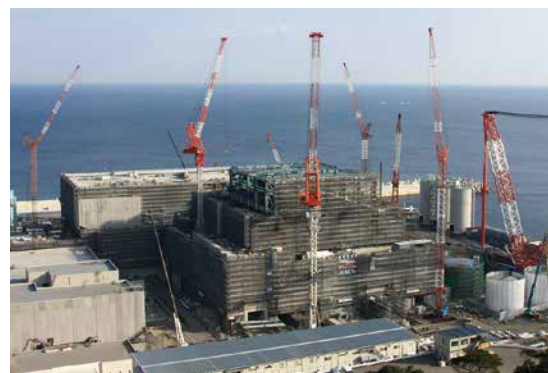
Shimane Nuclear Power Plant Unit 3 construction (as of February 2010)
