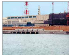
Kashiwazaki-Kariwa nuclear power station
