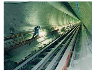
Kannagawa hydropower station
