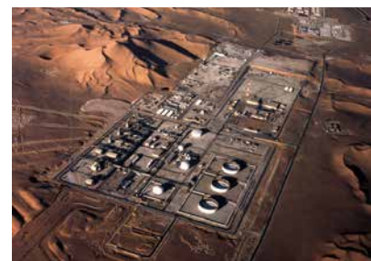
Natural Gas Facility
